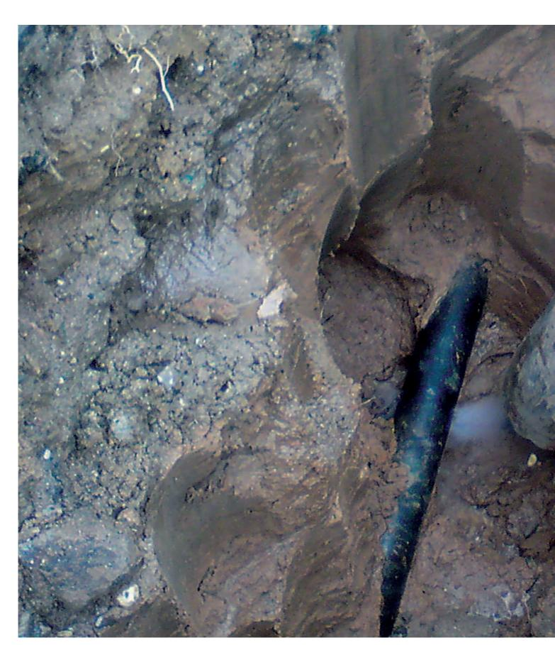
The pinpoint accuracy of our efficient suction technology means that the size of the construction trench can be reduced. This in turn reduces the amount of backfill and surface materials required, which has a considerable positive impact on overall repair costs.
