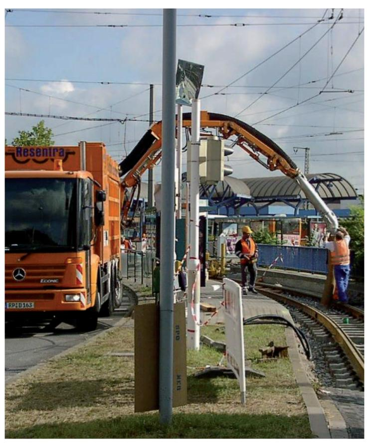
the intermediate spaces to do its job properly. This cleaning work can be carried out efficiently with a suction excavator. RSP even offers a two-way drive system solution designed specifically for this purpose.
